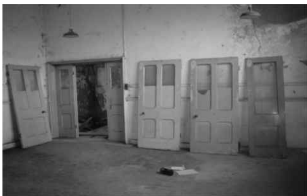
A number of doors have survived which can be reused. The door screens, shown here, and the classroom folding doors will also be restored.
