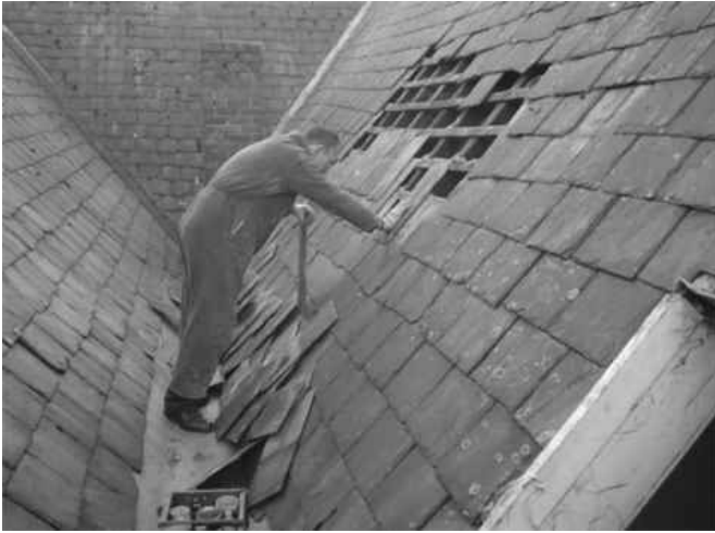
Autumn storms caused some damage to roof slates. It was impossible to find a roofer able to help so Trust Volunteers, John French and Ian Wolseley tackled the job, replacing dislodged slates. Other work completed by Friends John Walker, Jenny Watson and Vikky Lister has included tidying the site and clearing vegetation.
