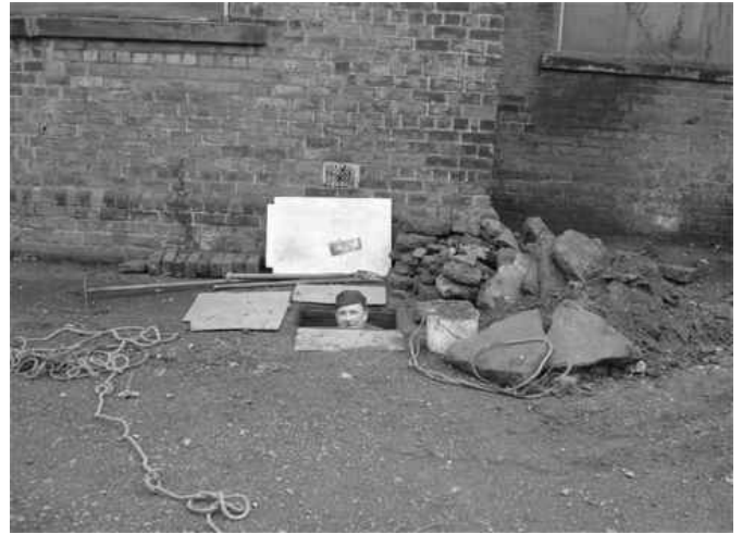
John French—up to his neck as usual—clearing a drain inspection hole. With the help of Friend, Martin Watson, the roof drains were kept clear during the recent heavy rains, and the ground drainage flows were monitored. Contractors jet-washed the drains and surveyed their condition using remote CCTV. It seems some of the original drainage will be re-useable.
