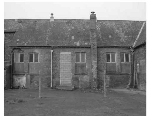
During the autumn the windows were unblocked to air and dry the building, and get light inside for internal works. Minor repairs to the roof were done too. Asbestos was removed and the site cleared of debris including thirty years of pigeon guano! The building was then pigeon-proofed.
